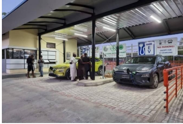
Figure 6.2: EV Charging station at UDUS,
