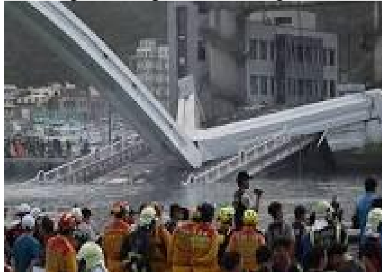
Fig 11 Pedestrian Bridge Collapse
